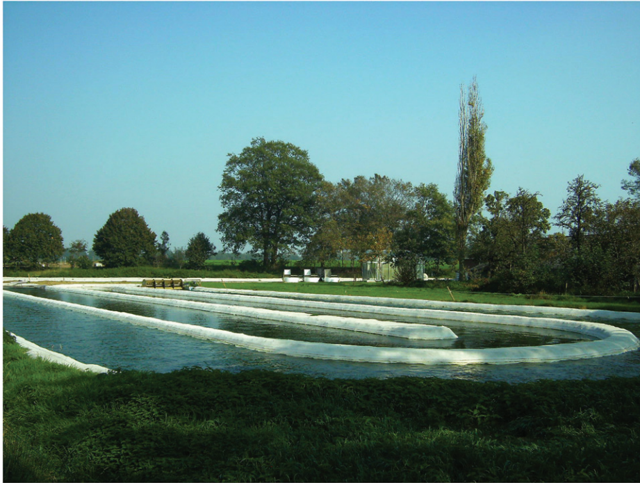
Figure 6. A raceway pond for the production of photosynthetic microorganisms. A paddlewheel circulates the water, exposing the microorganisms to uniform light and promoting rapid growth. Photo (online at Wikipedia) by JanB46, Creative Commons Attribution-Share Alike 3.0 Unported License.
